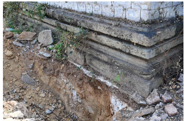
Original moulded stone base surviving below later masonry
