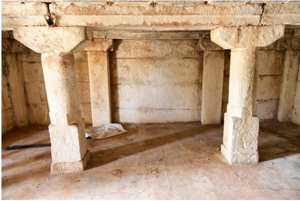
Interior pillars and beams before dismantling
